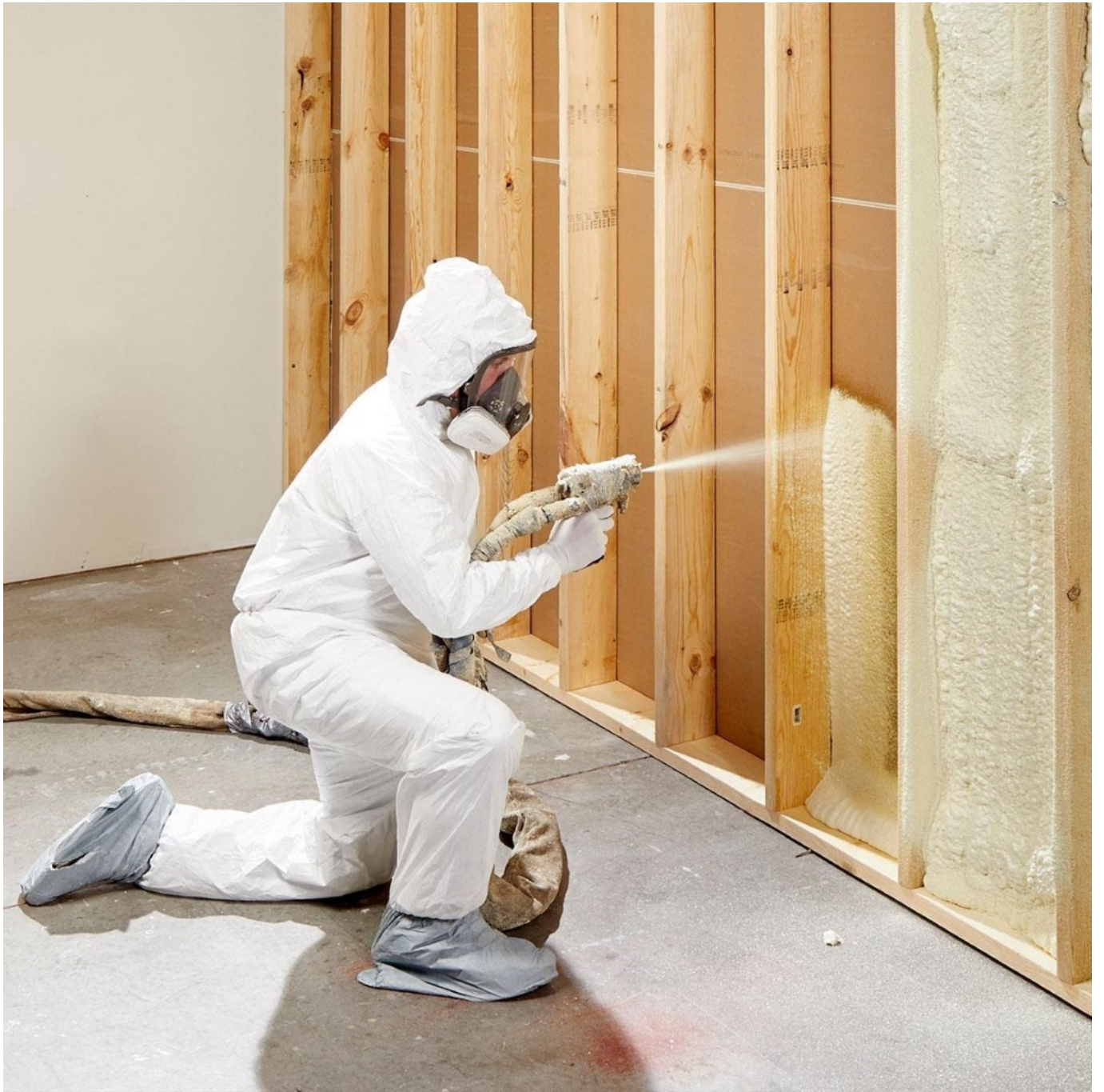
2 Part Foam Insulation- How To Work With It In Colder Temperatures
